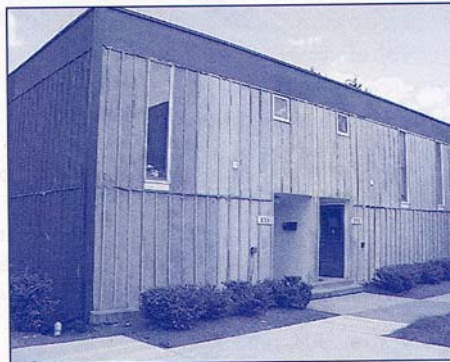
One hundred and one of the units are subsidized by a project-based Section 8 contract. The remaining unit is "market rate" but is restricted to residents who earn less than 60 percent of the area median income).
